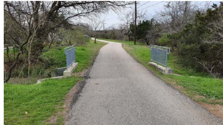
Leon Creek Greenway Trail Culvert
